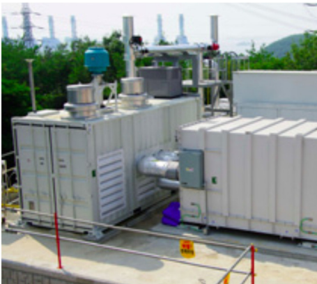
DFC@300 EU MCFC-Fuel Cell Power Plant 300 kW; 400 V; 50 Hz
